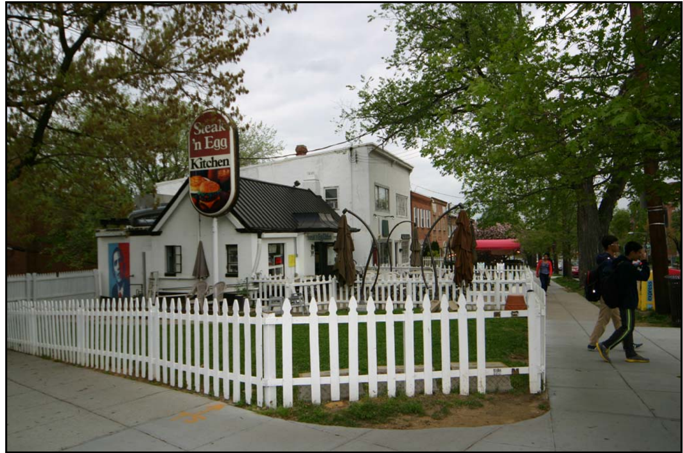
CORNER VIEW- CHESAPEAKE ST. & WISCONSIN AVE.
